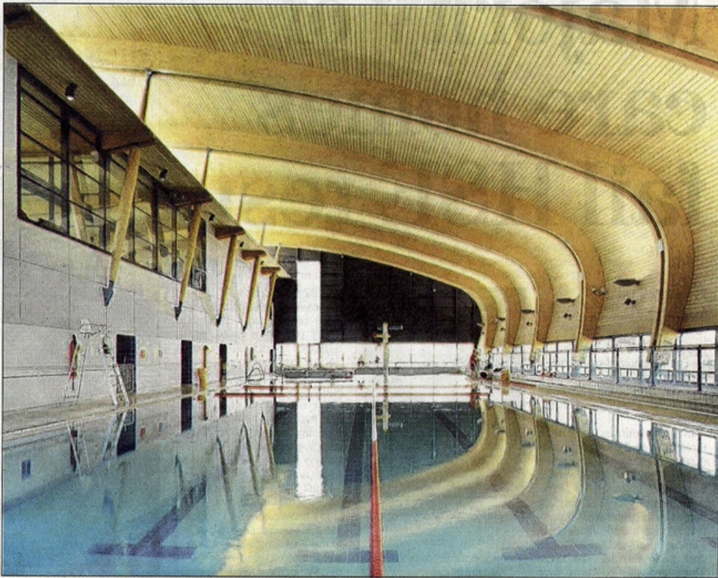
The design of the €7.2m Drogheda pool consists of two overlapping curved structures, with a roof that maximises natural light
