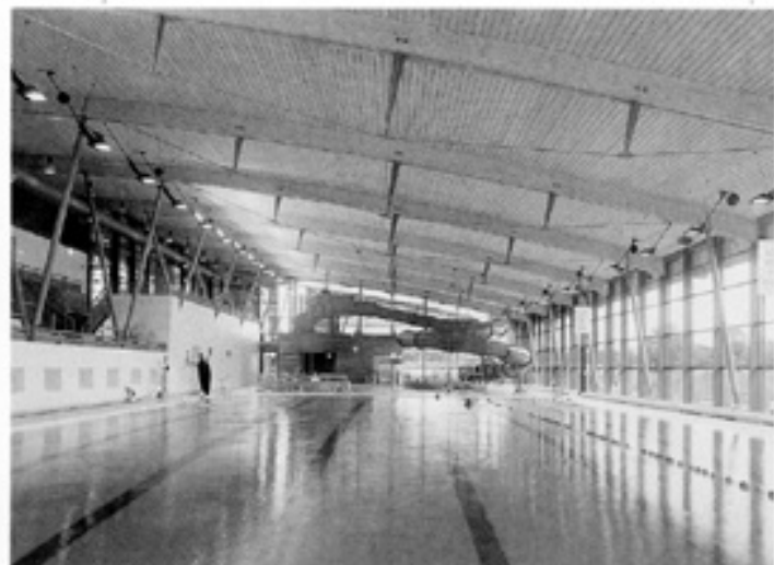
Blick in die Schwimmhalle | View of the swimming pool
